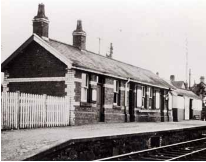
Hen adeilad gorsaf Y Groeslon // Former station building at Y Groeslon
