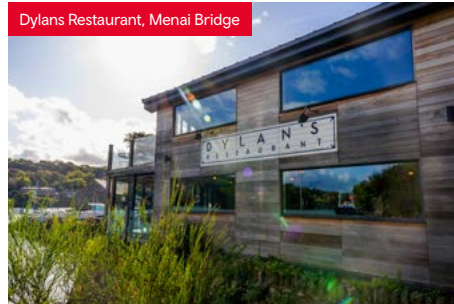
Dylans Restaurant, Menai Bridge
