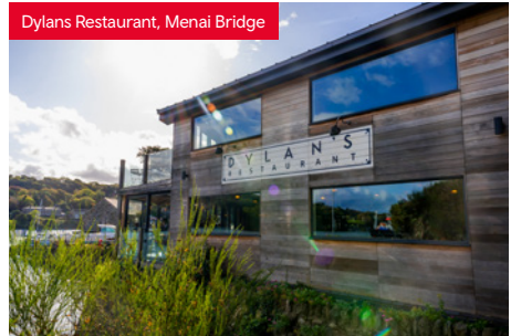
Dylans Restaurant, Menai Bridge
